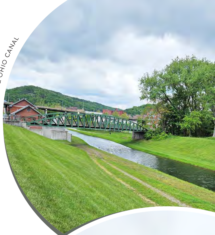
13 CANAL ST, WESTERN MARYLAND RAILWAY STATION
