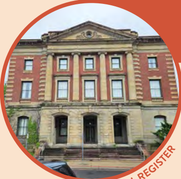
U.S. POST OFFICE BUILDING
