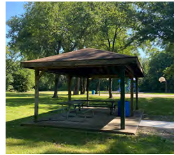
Picnic Shelter Fair condition
