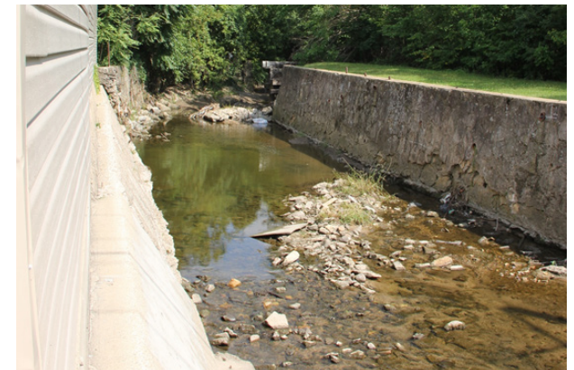
Concrete channel sidewall built into existing foundation at 2233 18th Street.
