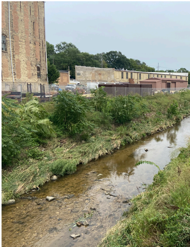
Old industrial buildings near 7th Street and Railroad Avenue
