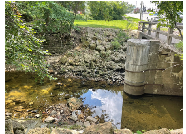
Sewer Manhole Located Adjacent to Bridge along Keith Creek
