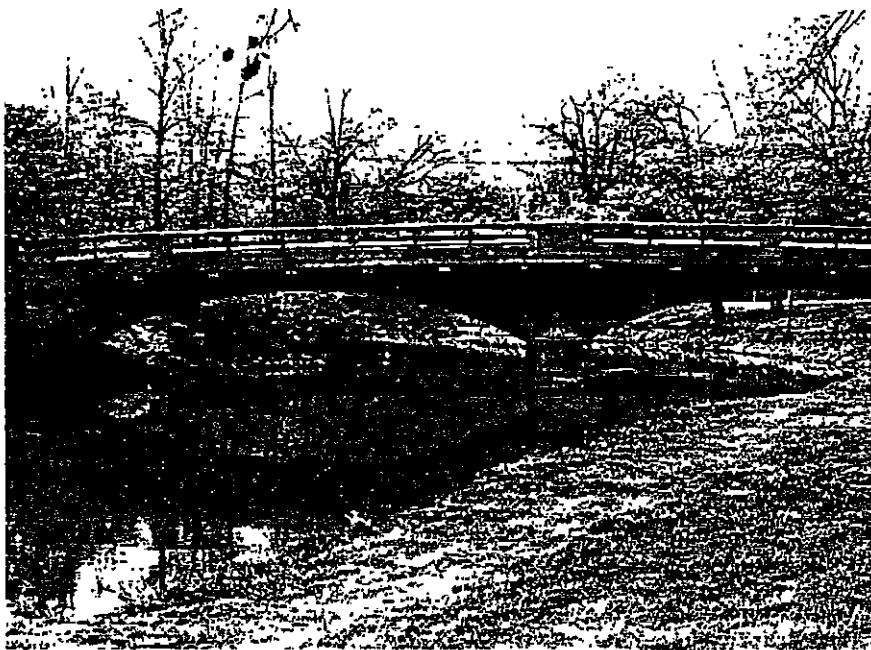
Figure 28: South entrance bridge to Island Park
