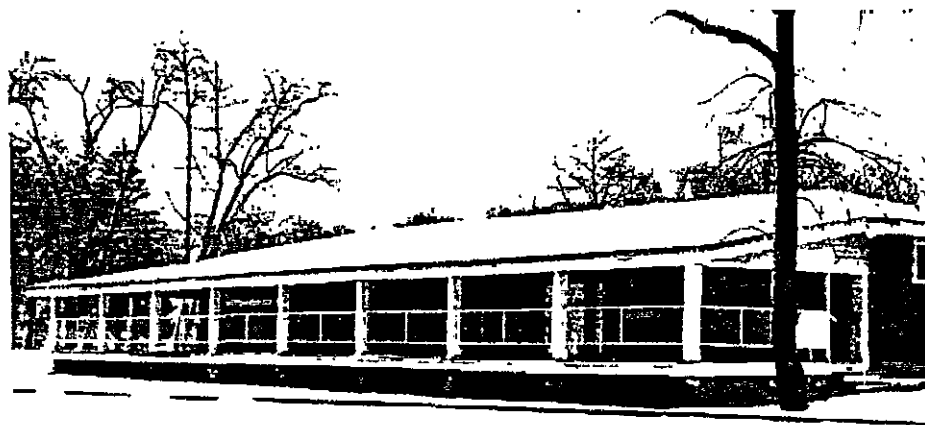
Figure 30: East facade of Refectory, Island Park
