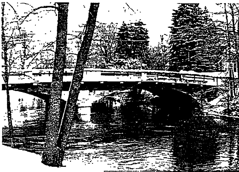
Figure: 29: East entrance bridge to Island Park
