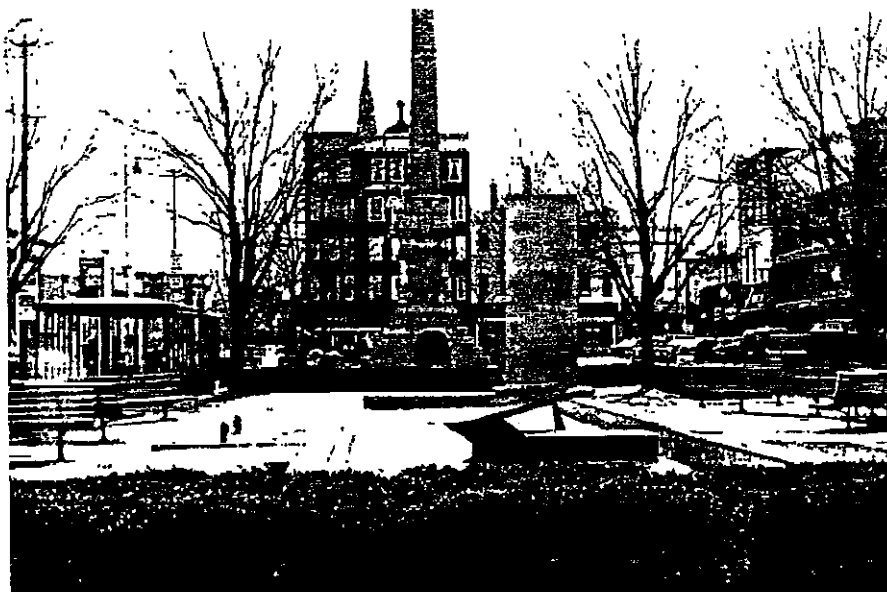
Figure 42: Monument Square looking north
