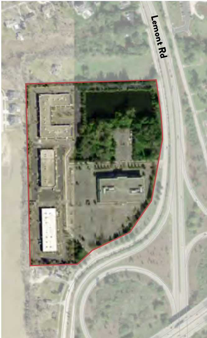
Figure 41: Lemont Road and I-55 Existing Conditions
