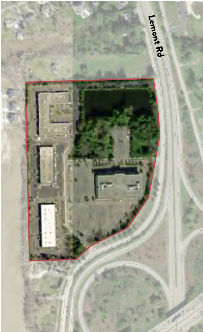
Figure 41: Lemont Road and I-55 Existing Conditions
