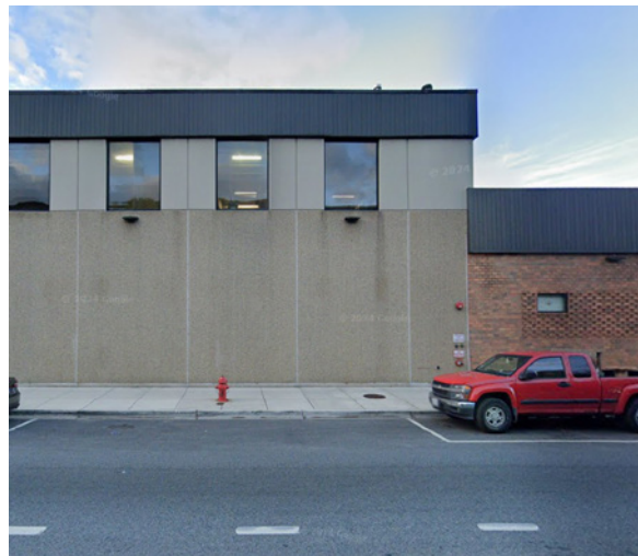
Industrial Character Area
