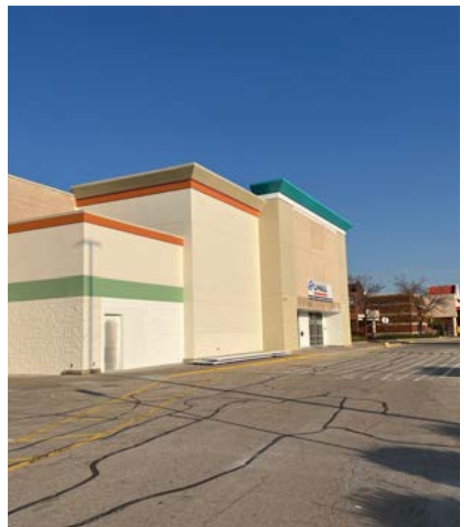
U-HAUL FACILITY, CENTERPOINTE
