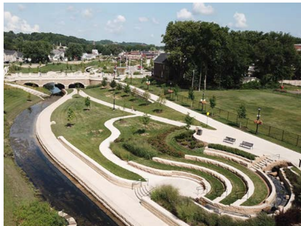
STEPPED STONE OUTCROPPING, BEE BRANCH
