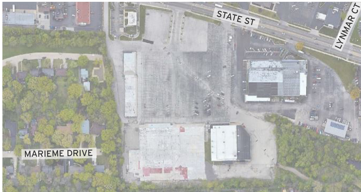
SITE EXISTING CONDITIONS
